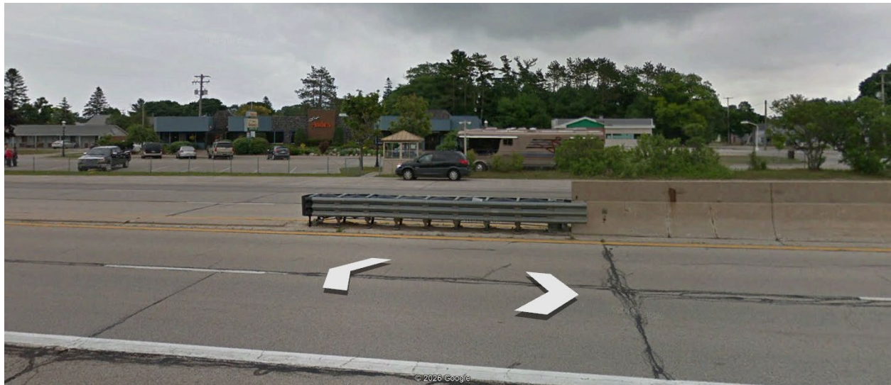
Southbound looking east at Existing Attenuator
