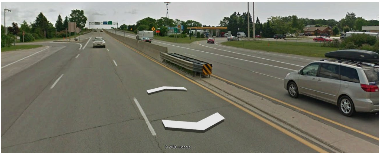
Northbound looking south at Existing Attenuator
